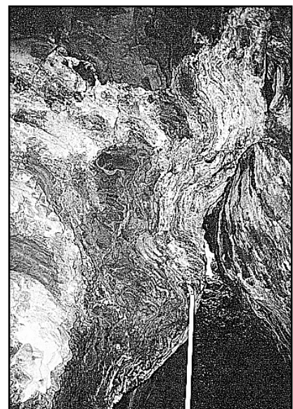
Figure 4: "Edge enhanced" detail of contorted wall linings near section X3. Staff is about 2m long.
