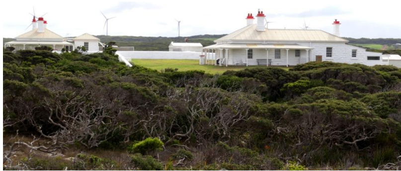
Lighthouse Keeper’s cottage & PV buildings
