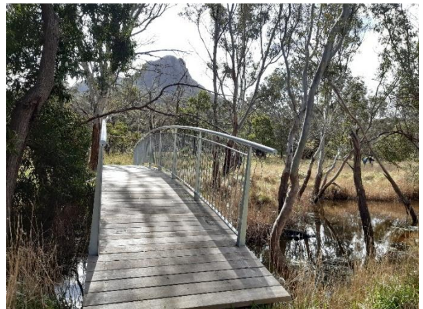
One of the new bridges over the Wannon River – Mt Sturgeon in the distance
