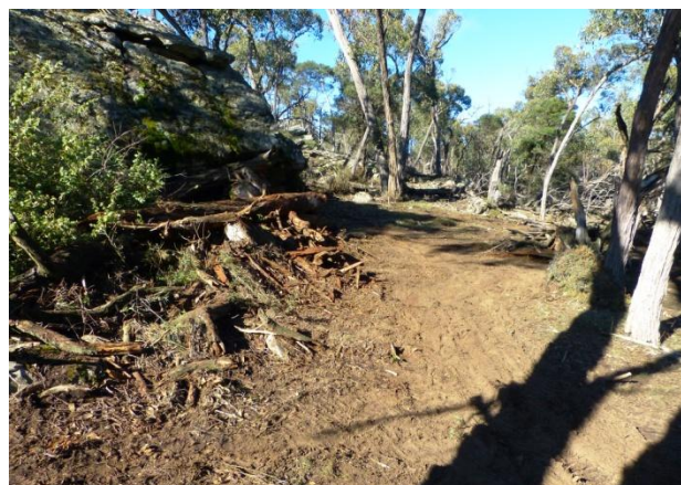
Clearing far S th on west side of range
