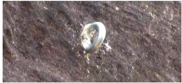
One of the bolts installed by climbers
