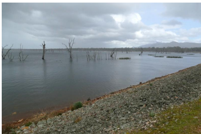
Lake Fyans looking south from levee bank
