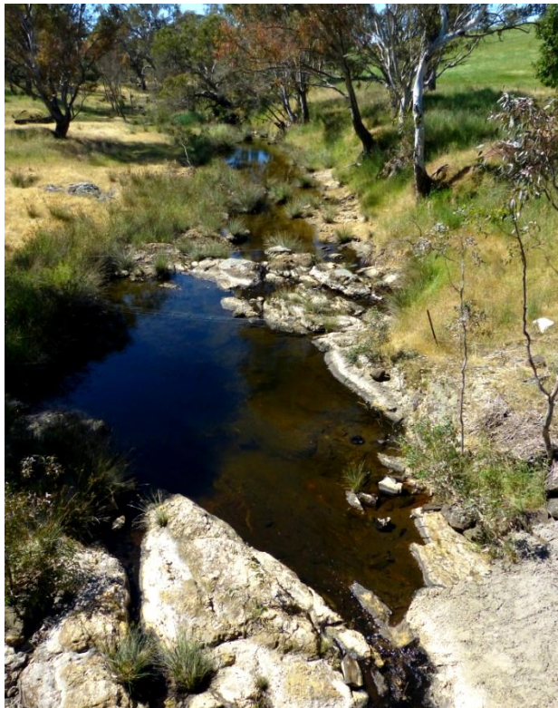
Stop 6. Yarramyljup Ck bridge on Balmoral Rd
