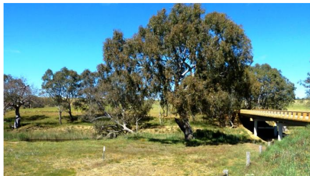
Stop 1. Red Gums & bridge over Hopkins River
