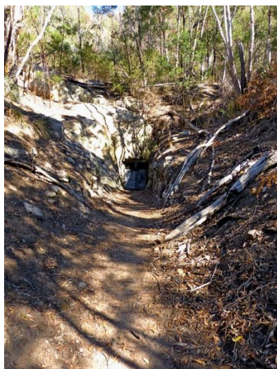
East end of Pomonal Tunnel
