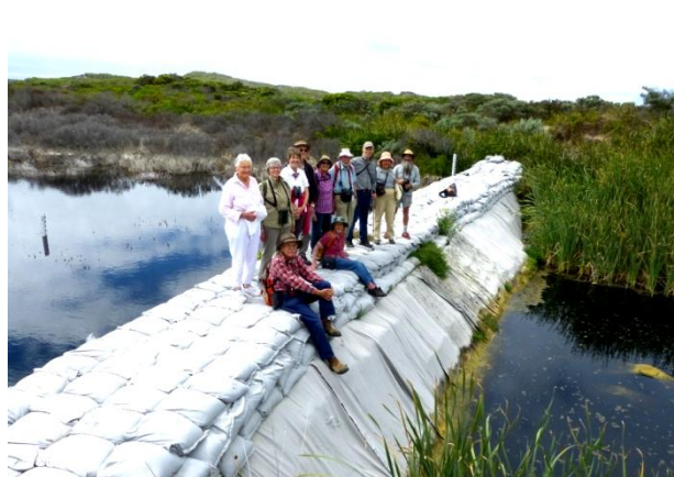
Phase 3 levee, Long Swamp – HFNC group.
