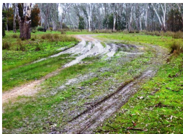
Off-track driving due to poor road condition
